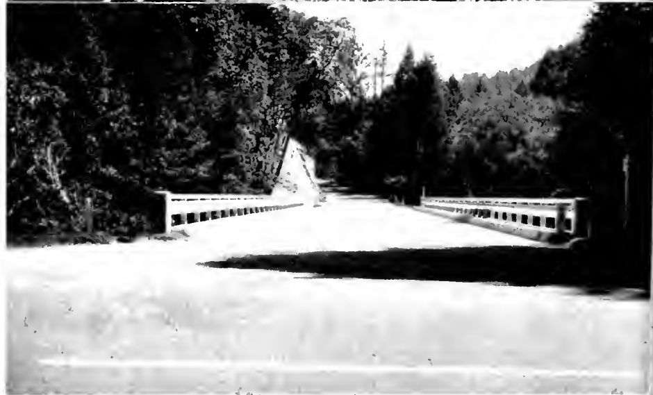
UPPER: Old San Lorenzo Bridge on Bear Creek Road in Santa Cruz County near the town of Boulder Creek. LOWER: New San Lorenzo River Bridge constructed by Santa Cruz County under the Federal Aid Secondary Highway Program.
